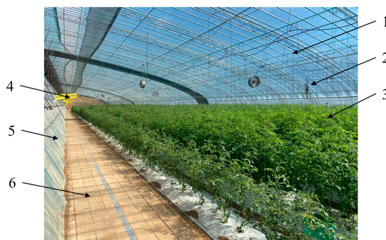
Figure 1. Schematic diagram of northern sunlight greenhouse cultivation for the experiment: 1: main skeleton; 2: greenhouse roof; 3: tomato plant; 4: north wall; 5: side wall; 6: concrete walkway.
