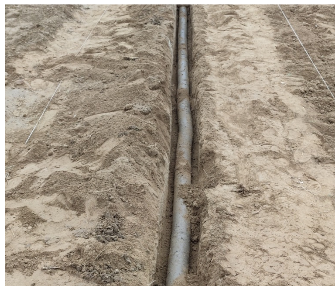
Figure 1. Stalk composite pipe placed in the trench.
