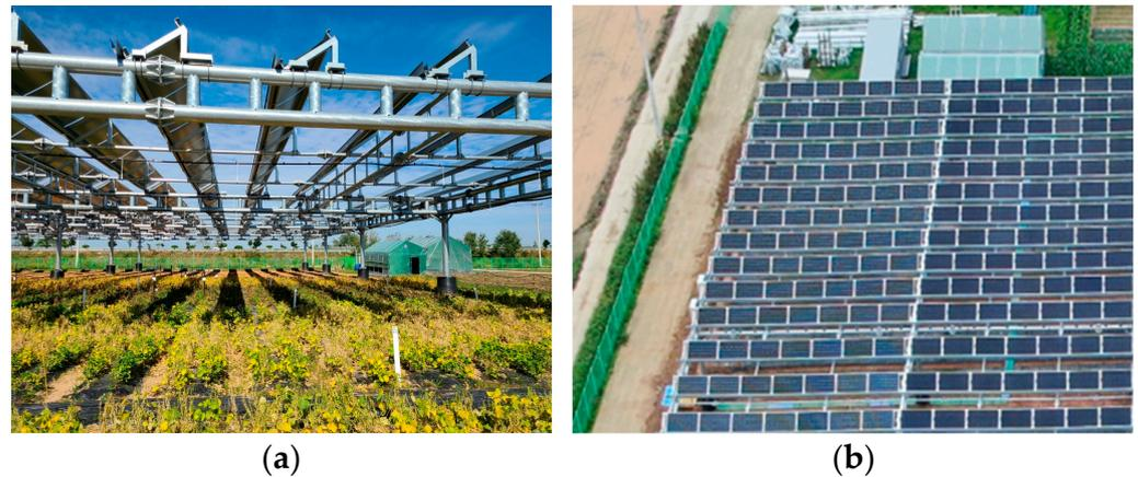
**Figure 1.** The agrivoltaic system in South Korea: (a) crops underneath photovoltaic modules; (b) photovoltaic modules.
