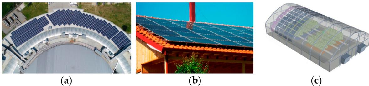
**Figure 2.** The roof building integrated photovoltaics (BIPVs): (a) rooftop PVs; (b) roof attached PVs; and (c) roof integrated PV.
