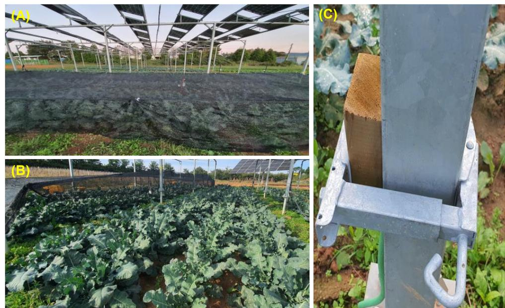
**Figure 2.** Photos of the west (A) and south side (B) agrivoltaic structure with additional shading in this experiment and bracket for installing shading net (C).
