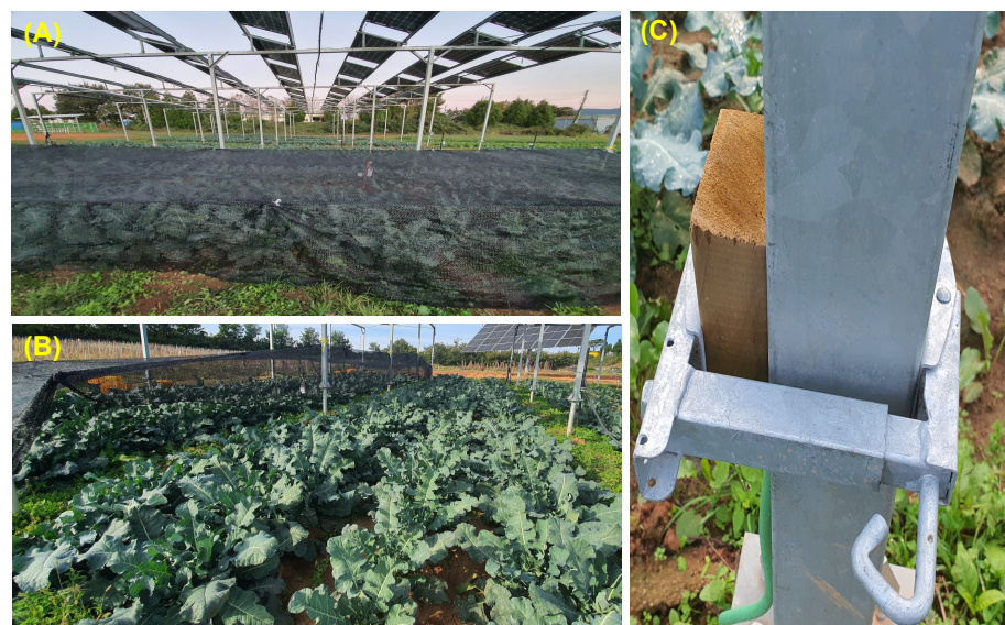
Figure 2. Photos of the west (A) and south side (B) agrivoltaic structure with additional shading in this experiment and bracket for installing shading net (C).
