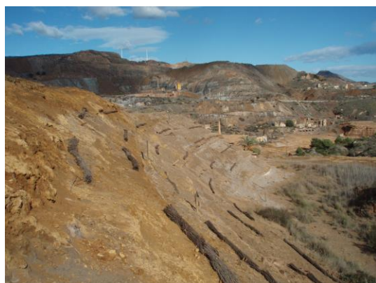
Figure A11. Detail of stabilization of slopes with heather sashes in Case Study 1.
