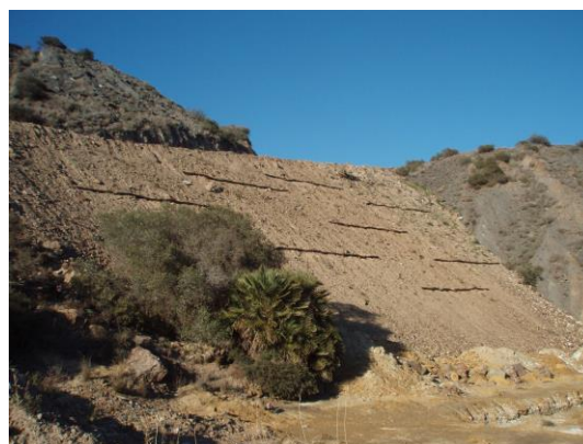
Figure A11. Detail of stabilization of slopes with heather sashes in Case Study 1.
