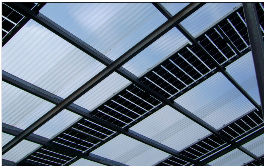
Figure 2. Example of producing solar energy inside the farm: innovative photovoltaic modules used as greenhouse cover material [37].
