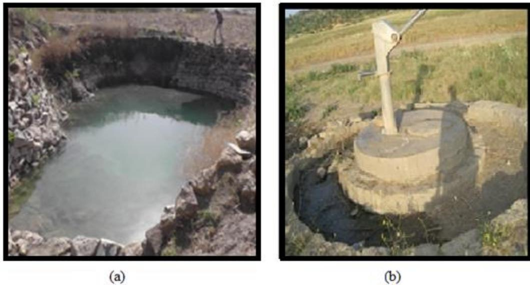
**Figure 5.** Some of the existing opened hand-dug well (a) and closed hand dug well (b) in the effective watershed area.
