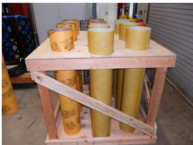
**Figure 6.** Wooden framework for column construction.
