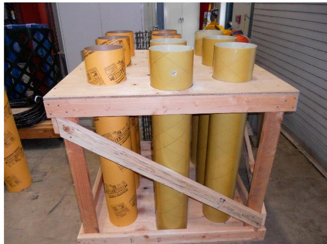
**Figure 6.** Wooden framework for column construction.
