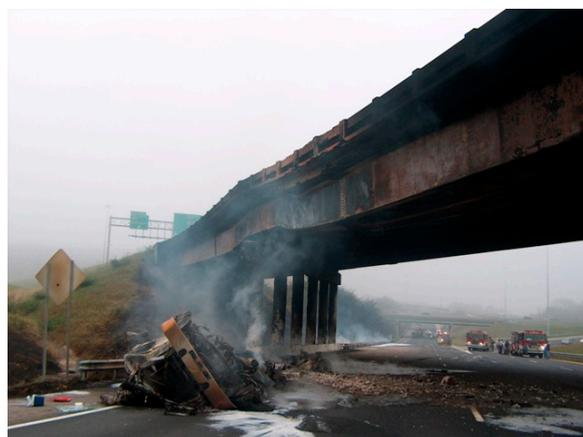
**Figure 1.** Visible bridge damage due to vehicular fire.
