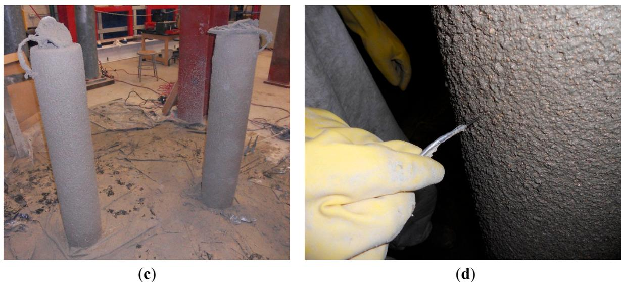
**Figure 8.** Complete process of Tyfo® CFP fire protection system application: (a) VG primer application; (b) VG dash coat application; (c) WR-AFP application; (d) thickness check of system.
