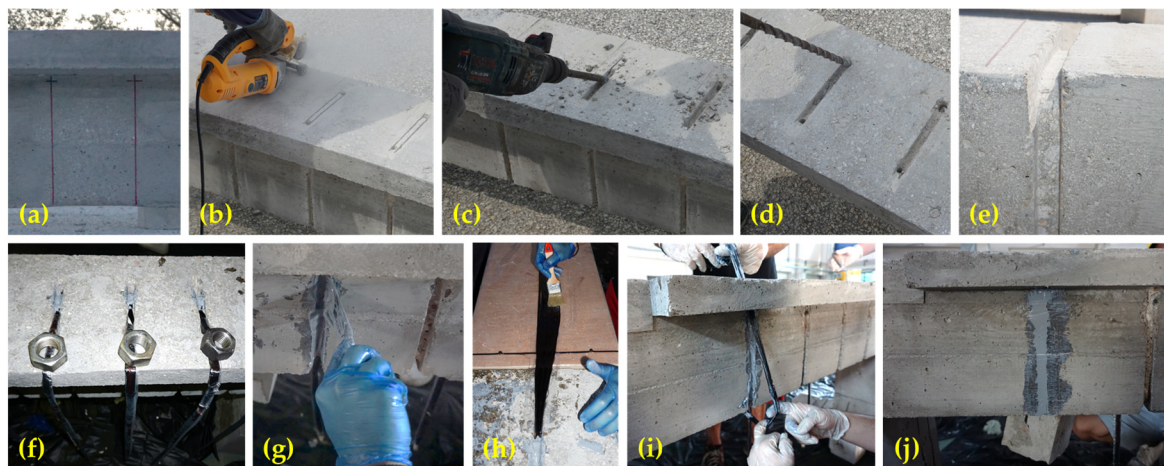
Figure 6. Step-by-step process of creating a closed-form stirrup using FRP rope in T-shaped RC beams (T-R150-W, T-R150-F, T-0.5R75-W, and T-0.5R75-F): (a) Marking retrofitting locations, (b) cutting notches, (c) drilling grooves, (d) drilling holes to connect grooves, (e) rounding edges, (f) impregnating and fixing a small portion of the rope end, (g) coating grooves with anchoring resin, (h) impregnating the remaining rope, (i) installing the rope, and (j) applying a small load for rope stretching and filling up grooves with resin.
