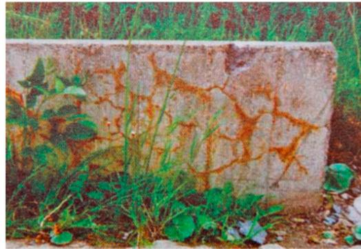
**Figure 11.** Map cracking due to alkali silica reaction, ASR deterioration on a concrete wall [94].
