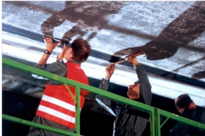
**Figure 1.** Application of externally bonded (EB) fiber-reinforced polymer (FRP) strip on Ibach bridge near Lucerne in Switzerland in 1991, what is believed to be the first application of EB FRP in the world (reproduced from [4]).
