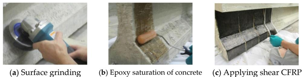
**Figure 4.** (a–c) EB FRP installation (reprinted from [24]).
