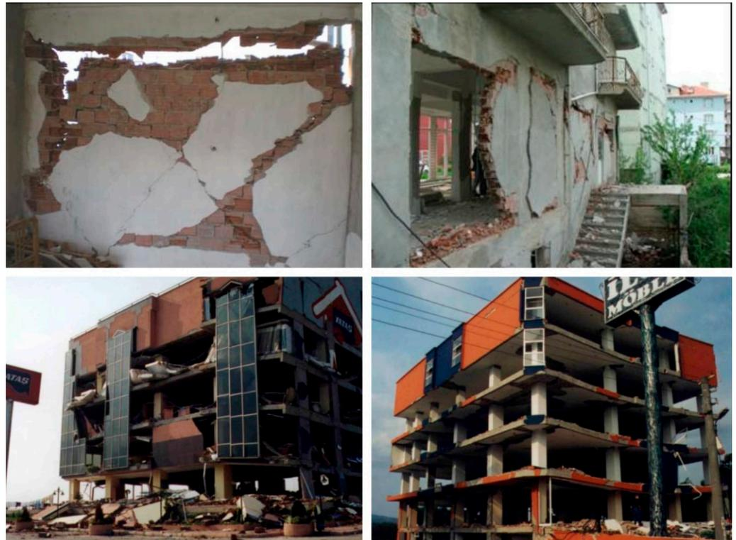
**Figure 1.** Infill wall damages from Simav, 2011, (top) [5] and Kocaeli, 1999, (bottom) [4] earthquakes.
