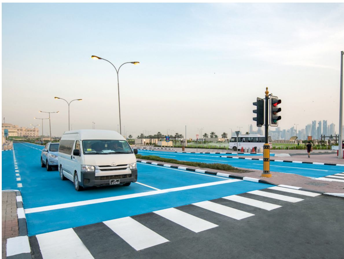
Figure 6. The implementation of a pilot scale for cool pavement paint is underway on Abdullah Bin Jassim Street [76].
