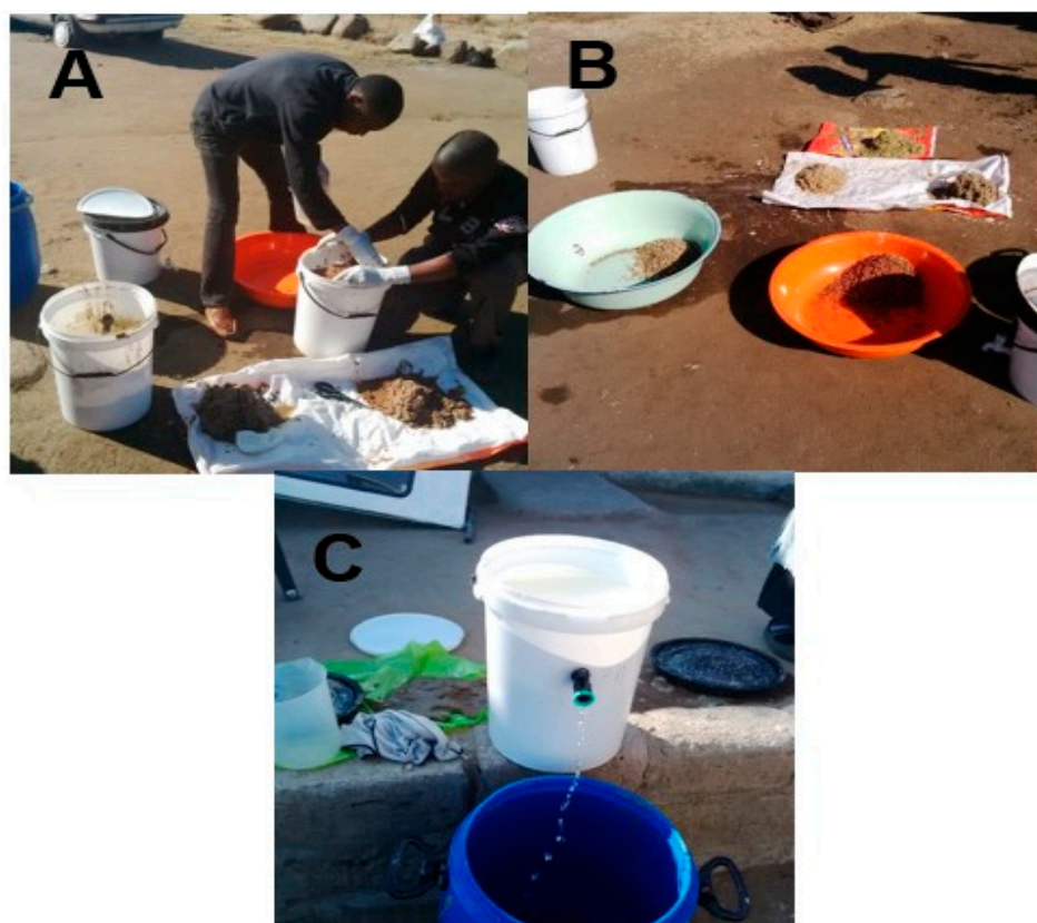
Figure 3. Maintenance of the BSZ-SICG filter implemented in Makwane Village. (A) Training of one of the householders on how to wash the layers of the BSZ-SICG filter; (B) all five layers after being washed (gravel, coarse sand, fine sand, natural zeolite, and silver-impregnated clay granules); and (C) filtered water after the washing of the BSZ-SICG filters.
