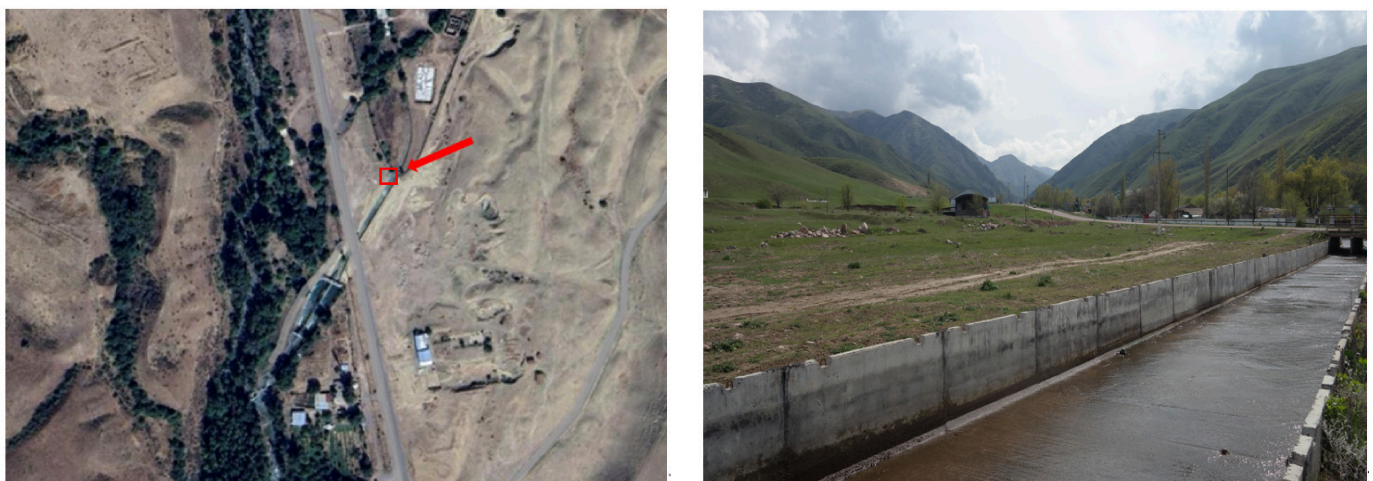
Figure 3. Installation location system for testing the system on the Merke River.
