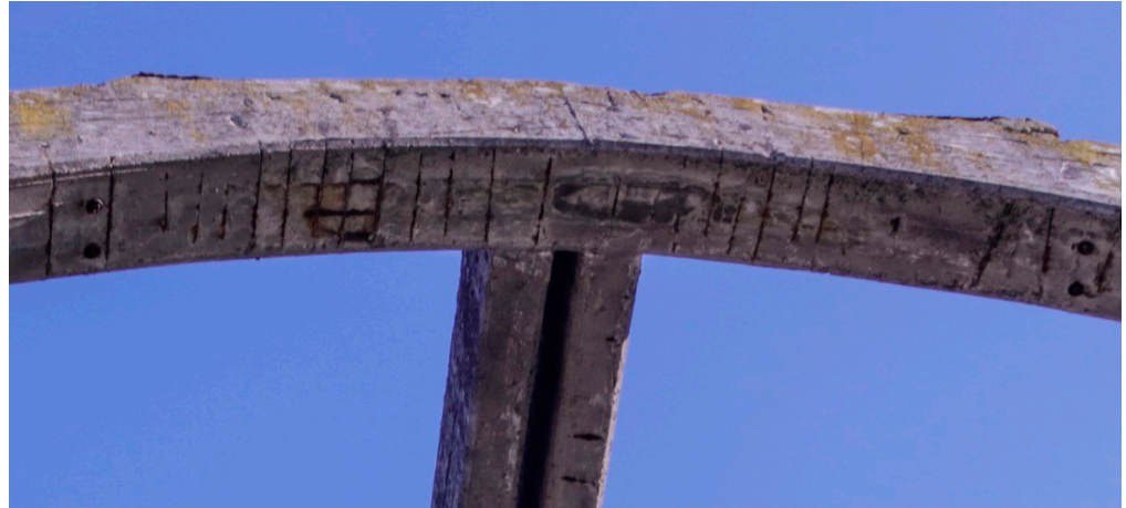
Figure 9. Example of exposed iron located in the intrados of the concrete arch.
