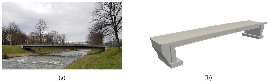
**Figure 6.** An image of the bridge used in this study in (a). Pedestrian bridge over the Dreisam river in Freiburg, Germany with a length of 40 m. The model of the bridge obtained from [18] can be seen in (b). Parts of the bridge's foundation are not visible as they are located underground.
