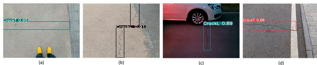
**Figure 11.** Outcomes of YOLOv5-based road crack detection: (a) Road crack I; (b) Road crack II: shadow; (c) Road crack III: dark light; and (d) Road crack IV: lane line.
