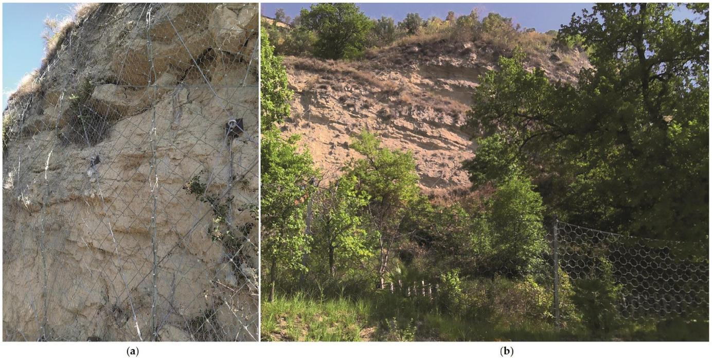
**Figure 6.** Example of rockfall barriers: rockfall protection net in Monte San Martino (a) and rockfall protection fence in Montefalcone Appennino (b).
