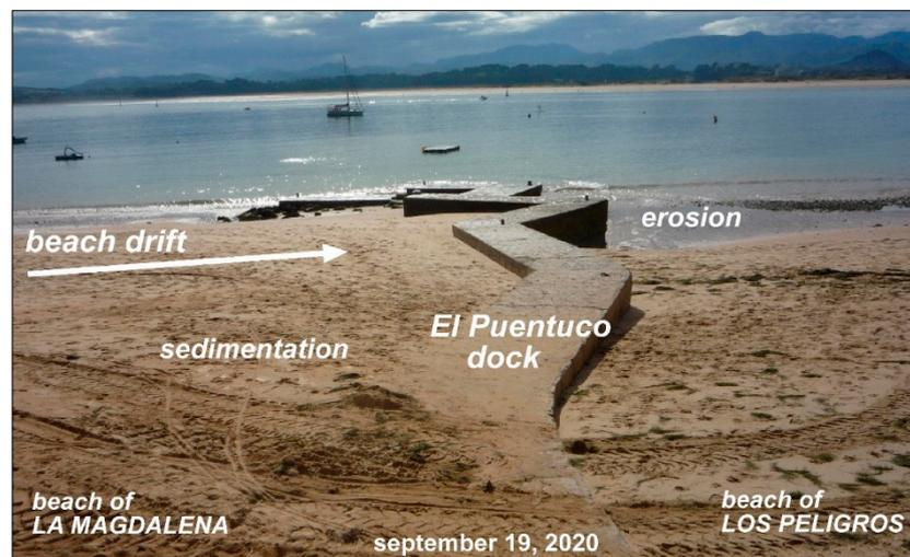
Figure 9. El Puentuco dock is situated at the dividing point between Zone 2 (La Magdalena) and 3 (Los Peligros). It has been covered by sand in the last decades and became visible in 2020 after the construction of the breakwater. Now, it retains part of the sand drift from La Magdalena.
