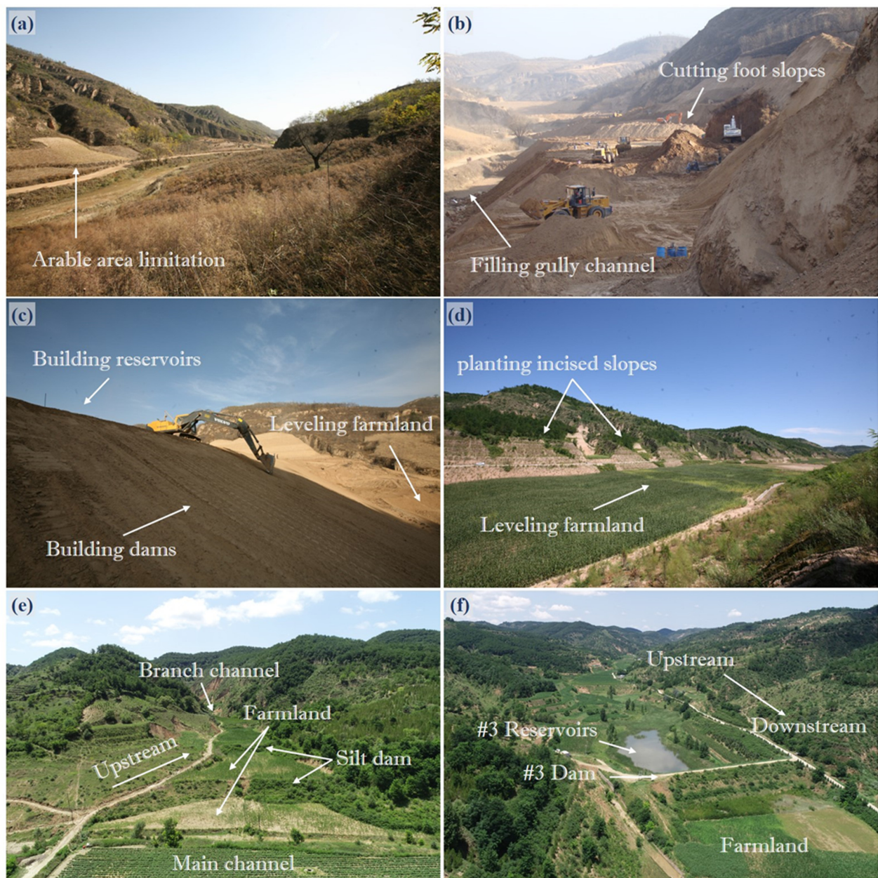
Figure 1. Site photos showing the process and local situation of the GLCP implemented in the Gutun watershed (GTW). (a) Original landform; (b) cutting foot slopes and filling gully channel; (c) building dams and reservoirs; (d) leveling farmland and planting cut slopes; (e) landscape of branch channel; (f) upstream landscape of #3 reservoirs and dam.
