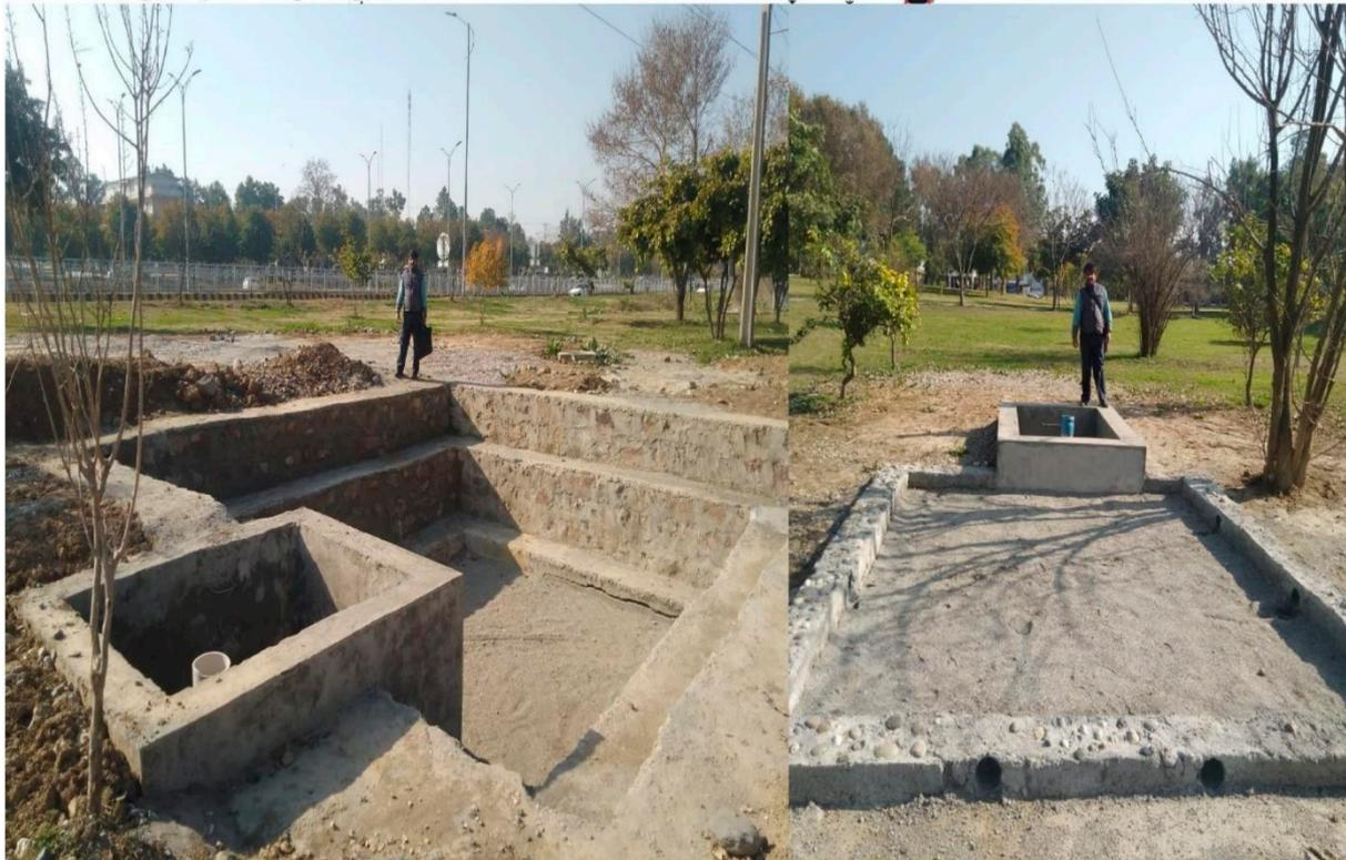
**Figure 11.** Technical design, coral design, and constructed recharge well on suitable sites.
