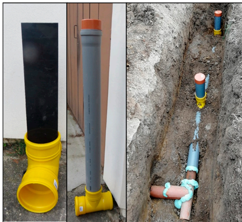
Figure 2. Underground fixed WLCS consisting of a drainage T branch (yellow), a polypropylene gate (black) and a PVC pipe vertically connected to the T branch (grey) with a cap (brick-red); before and after installation on tile drainage.
