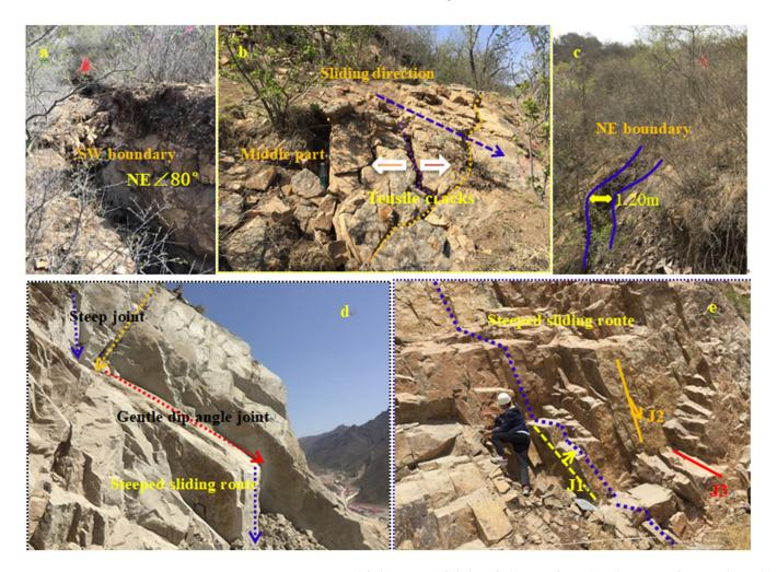
**Figure 15.** Composition and failure type of sliding failure surfaces (combination of stepped-gentle joints). Combination of stepped-gentle joints of sliding failure surface. (a) tension fissure at trailing edge. (b) tensile cracks in middle part. (c) shear fissure at NE boundary. (d) Combination of anti-inclined joint and inclined unloading joint. (e) Combination of inclined joint and inclined unloading joint.
