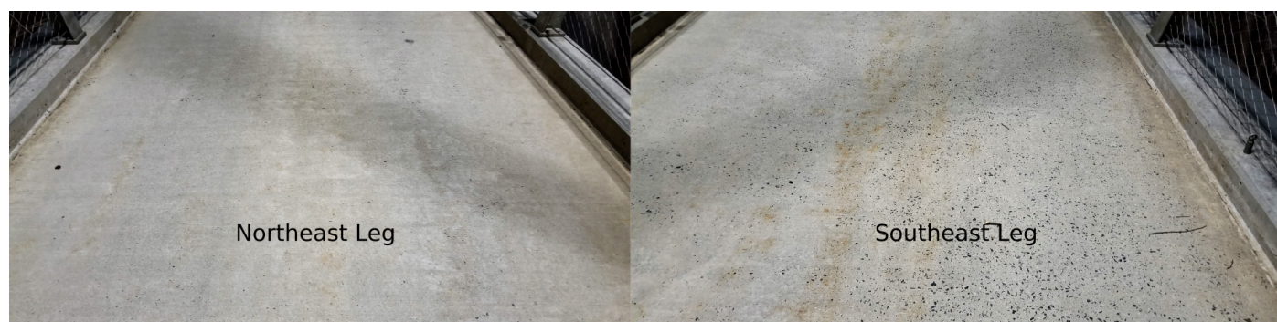
Figure 13. Figure showing increased loss of cover on the southeast leg compared to northeast leg.
