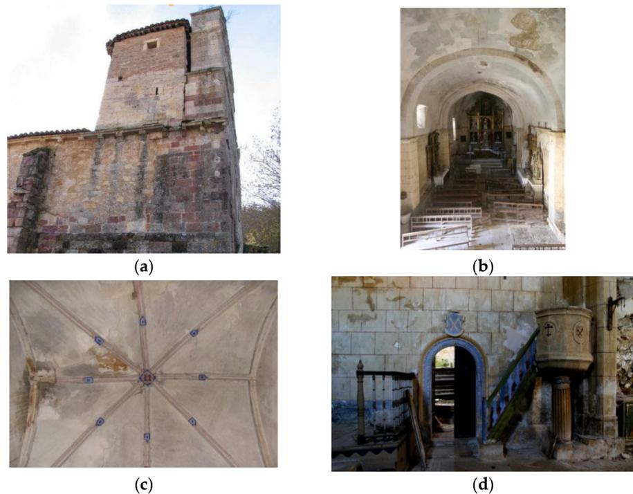
**Figure 3.** Conservation status before the intervention: (a) structural movement of the tower; (b) large deformation in the main nave; (c) cracks, moisture and detachment on the ribbed vault and (d) presence of moisture, erosions, detachment and garbage at the entrance of the annexed body.
