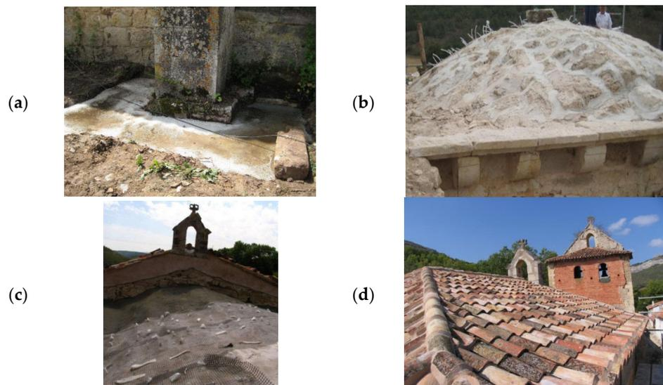
**Figure 4.** Restoration works at structural level: (a) addition of armoured concrete to one of the buttresses of the main nave; (b) preparation of the extrados surface of the ribbed vault for the application of the textile reinforced mortar (TRM) layers; (c) application of the TRM solution and (d) final appearance of the roof.
