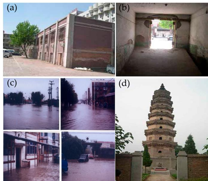
**Figure 1.** Hazards of land subsidence in Hebei Plain. (a,b) The Cangzhou People’s Hospital sank due to land subsidence. (c) Water accumulation caused by land subsidence in Cangzhou; (d) The Putong Temple tower skew caused by land subsidence in Nangong County, Xingtai City (provided by Hebei Geo-Environment Monitoring).
