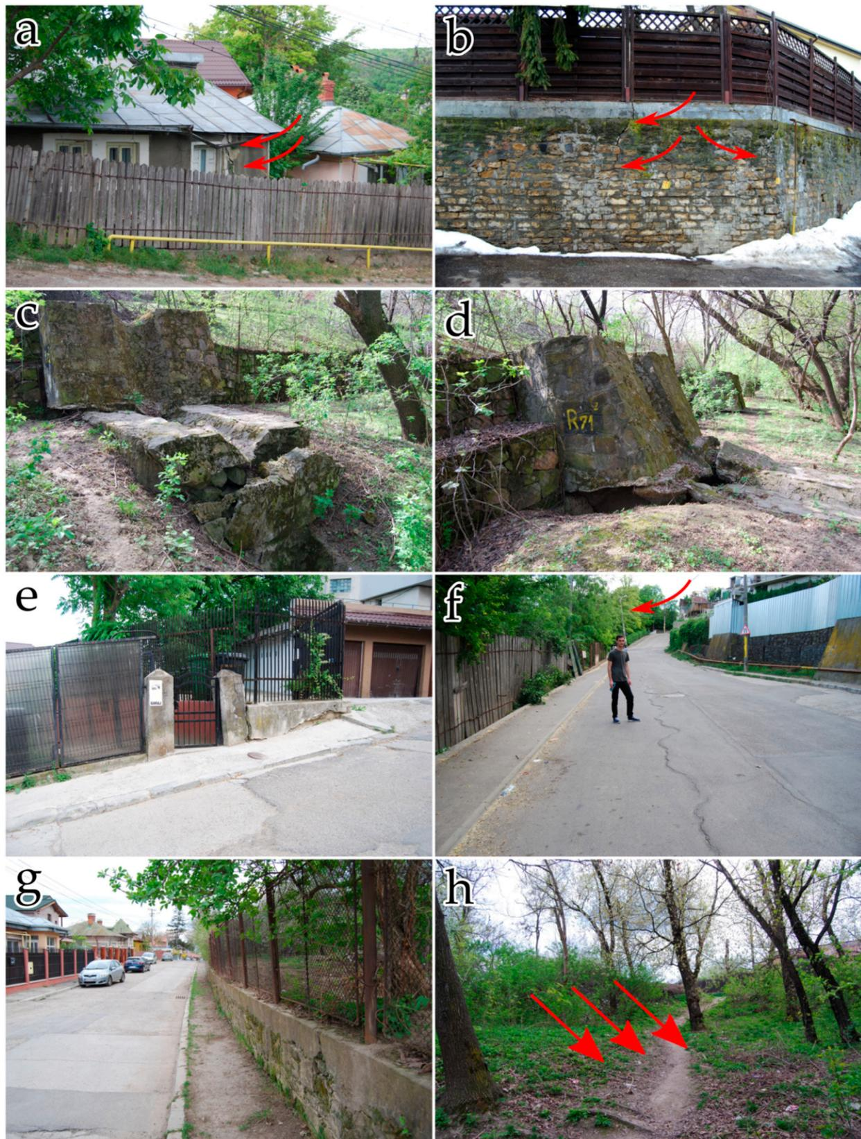
**Figure 4.** Evidence of surface displacements occurring over the Țicău landslide affected area. (a) Centimeter cracks in the outer wall of a house; (b) wall cracks; (c,d) damage to stabilizing infrastructure; (e) damaged fence; (f) roadway cracks and leaned electric pole (red arrow); (g) wall bulging; (h) tilted trees, red arrows indicate the direction of displacement. (high-resolution image available at <https://doi.org/10.6084/m9.figshare.14915250.v1>).
