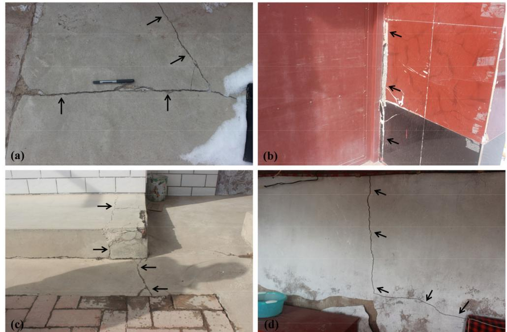
**Figure 14.** Field work photos showing some damage to roads and buildings caused by the tunnel excavation, where the black arrows indicate the cracks. (a) The damage to the road; (b) the damage to the building; (c) the damage to the road; and (d) the damage to the building.
