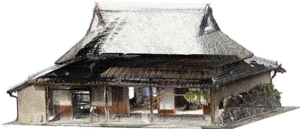
**Figure 4.** The 3D laser-scanned data of the former Nakajima Residence, which is a traditional Southeast Asian folk house (24,074,424 points).
