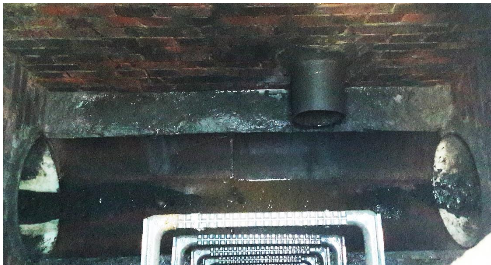
Figure 17. Visual inventory of a sewage drain with visible main string and transverse connection.
