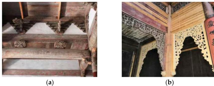
**Figure 2.** The repaired Huizhou-style buildings of timber components in the (a) JiXi Confucian Temple (which had been historically repaired and restored three times during Qing dynasty) and (b) Chengzhi Tang in Hong Village HuangShan, Anhui Province.
