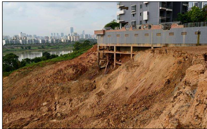
Figure 3. Example of the heavy damages on building caused by the Liusha Peninsula landslide on 12 July 2014.
