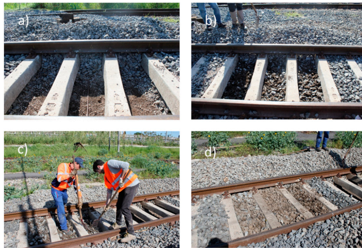
Figure 3. Preparation of a single sub-section within the test-site area; (a) a set of three slots is emptied out of the original ballast; (b) the slots are filled up again with the test material; (c) the material is arranged and compacted in order to fill all the voids; (d) the re-arranged configuration.
