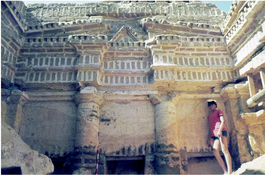
Figure 3. Qasrawet #1137, Site D50 (Anomaly #1). South face of the central temple's inner structure. Engaged columns crowned by square capitals, topped by a heavy wooden beam (entirely decayed) which supported the Egyptian style cornice and above it a gable with dentils inside a broken pediment (Photo E.D. Oren).
