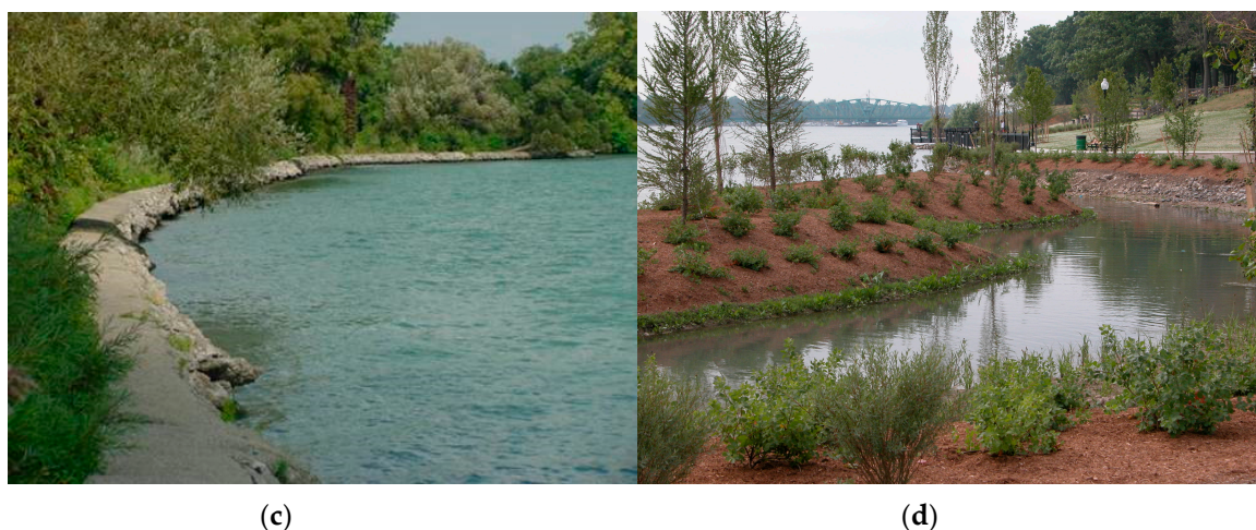
Figure 4. Photographs of soft shoreline engineering projects at Rouge Power Plant in River Rouge, Michigan ((a): before and (b): after) and Wayne County’s Elizabeth Park in Trenton, Michigan ((c): before and (d): after) (photo credits: Rouge Power Plant shoreline: Nativescape, LLC (Manchester, Michigan, USA); Elizabeth Park: U.S. Fish and Wildlife Service (Grosse Ile, Michigan, USA)).
