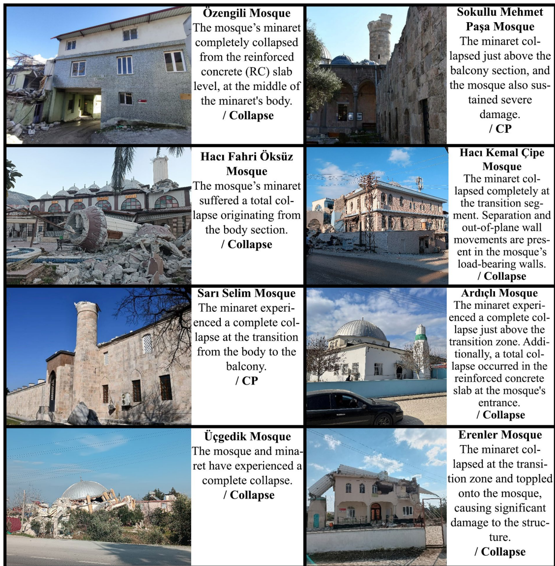
Figure 10. Earthquake-Induced Damages to Masonry and Reinforced Concrete Mosques and Minarets in Hatay (photos by the authors).
