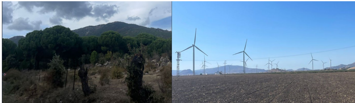
Figure 7. Alternative wind turbine installation locations in the Bergama region.
