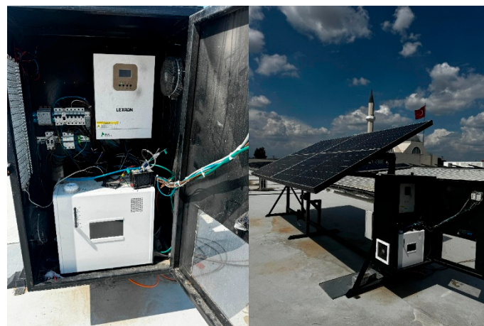
Figure 3. Solar Inverter Connection and System Overview.
