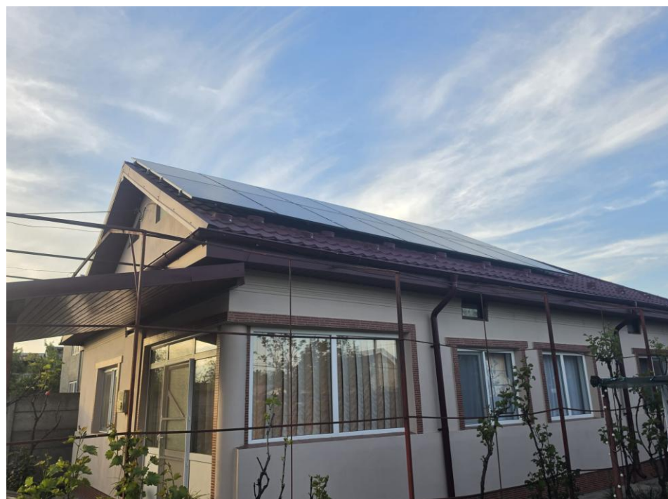
Figure 3. General view of the building.
