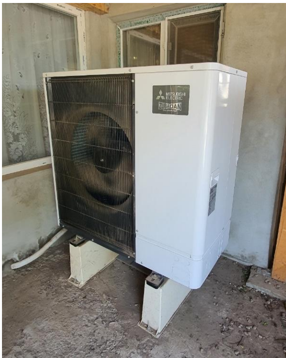
Figure 4. Front view of the air-to-water heat pump: (left) indoor unit; (right) outdoor unit.
