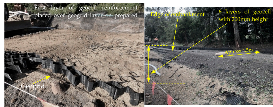
Figure 8. Construction of the temporary Wattamolla Road embankment using a six-layer geocell mattress system [1].
