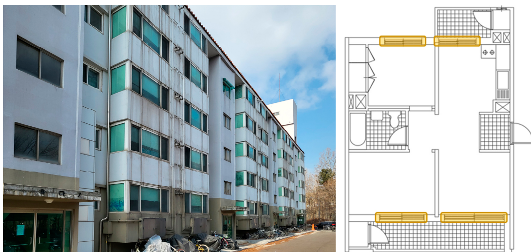
Figure 8. Picture and floor plan of the selected apartment building and the locations of the installed secondary glazing system highlighted in yellow.
