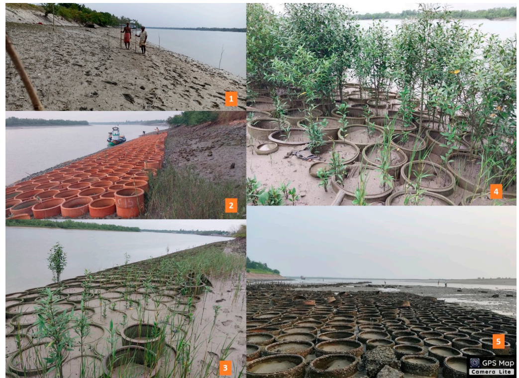
Figure 6. (1) Site 4 barren patch in front of the embankment, (2) terracotta silt trap installation, (3) emergence of mangrove species, (4) growth of Avicennia marina in silt traps, and (5) oysters in silt traps at Site 1.
