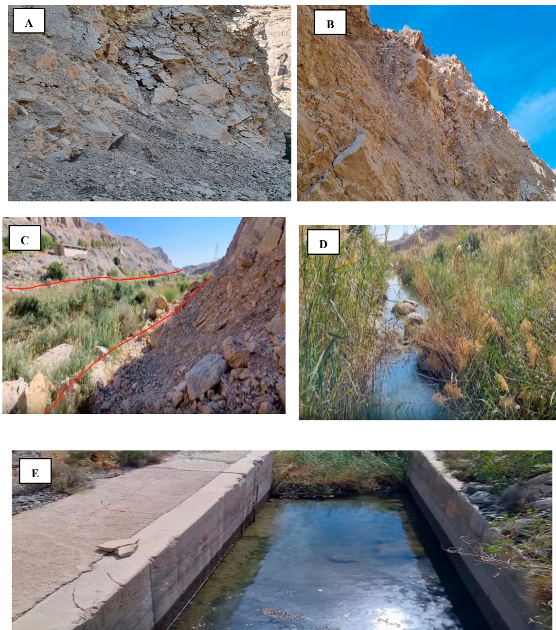
Figure 2. (A,B) The fracture and weathering zones along the Jiroft Dam path. (C,D) The position of the dam spillway channel among unstable areas. (E) The dam spillway channel runs parallel to the river and is connected to it through a curved path.
