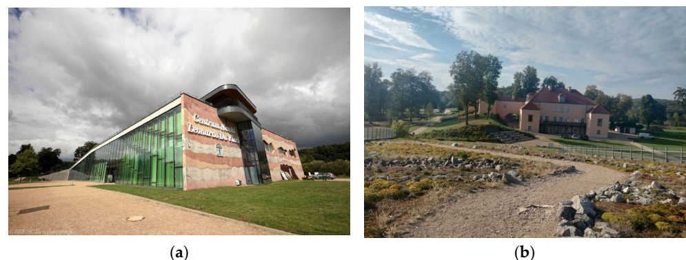
Figure 10. Podzamcze Chęcińskie. Leonardo da Vinci Science Centre. View of the building that fits into the area. (a) (photographs: Author Olga Cicha, Anastasiia Dubyna, 2025). View of the Palace. (b) (photographs: Author Olga Cicha, Anastasiia Dubyna, 2025).
