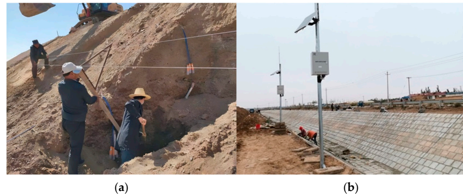
Figure 4. On-site installation of monitoring instruments. (a) Installation of monitoring instruments on canal slopes; (b) remote, automated data collection system.
