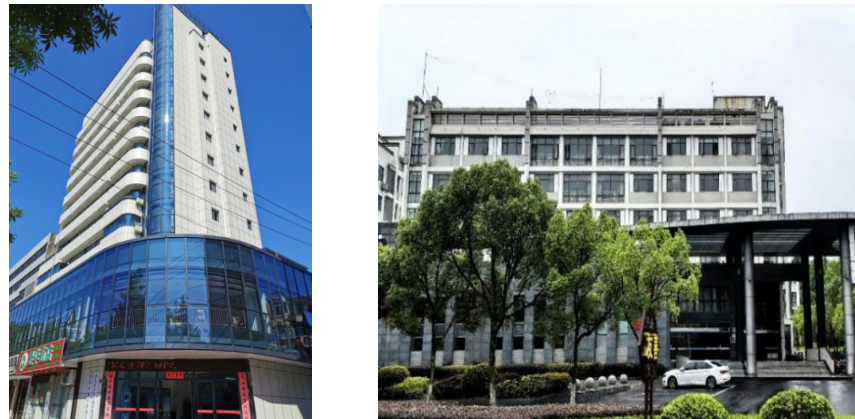
Figure 11. Facades of an office building in Huangshan and an office building in Shexian County.
