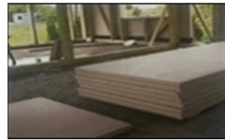
Figure 2. Compressed-straw panels. It is a building panel made of compressed straw covered with recycled cardboard. It is a stable, easy-to-process, and sound-insulating material.
